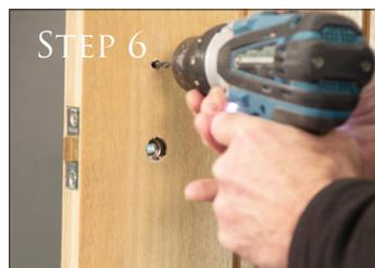
Once you have marked everything up drill a hole that goes the complete way through the door as in this how-to we will be using male to female bolt through fixings. Wood screws can be used just no need to drill all the way through the door. The bolt-through fixings give a much better result.
