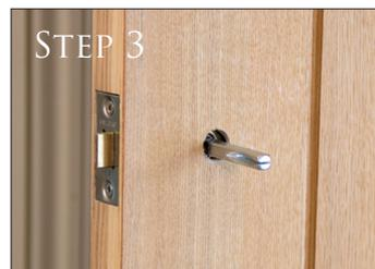
The spindle provided is designed to be used with a range of door thickness's so you may need to adjust the length depending on your door. You can check this by fitting the second handle to the other side of the door and seeing how much (if any) spindle is spare (still showing). Measure this amount and go to step 4.
