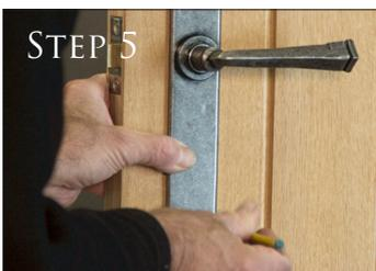
When you are happy with the fitting of both handles and the spindle length it is time to begin fixing the handles in place.
