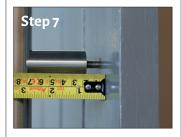
Using a tape measure check the amount which will need to be removed from the bolt.
