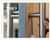
Locate the two grub screws underneath the fixing arms of the second handle and loosen. Place the handle over the ends of the grooved bolts and hold securely in place.
