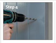
The next step is to drill the holes needed to fit the back-to-back fixings. So it may be a good time to double check everything is centered and positioned how you want it.
