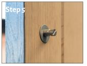
Once both holes have been drilled pass the bolt through the hole using the metal washer (if using on a glass door the rubber pads must be used first then the metal washers).
