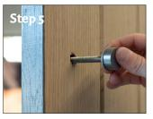
Once both holes have been drilled pass the bolt through the hole using the metal washer and bolt end (if using on a glass door the rubber pads must be used first then the metal washers).
