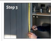
Depending on the length of handle chosen you need to check your fixing centre measurement and mark the lower point on your door.
