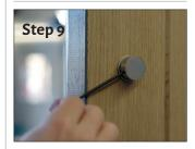
There is a small hole on each of the bolt heads where you can fit a allen key and begin to rotate the bolt to give that final tighten and create the perfect fit.
