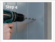
The next step is to drill the holes needed to fit the bolt-through fixings. So it may be a good time to double check everything is centered and positioned how you want it.
