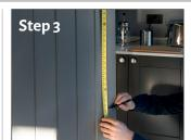
Depending on the length of handle chosen you need to check your fixing centre measurement and mark the lower point on your door.
