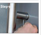
With the handle pushed tight against the surface of the door use the allen key to secure the grub screw onto the groove in the fixing sleeve.
