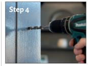
The next step is to drill the holes needed to fit the grommets that come with the secret fixings. So it may be a good time to double check everything is centered and positioned how you want it.
